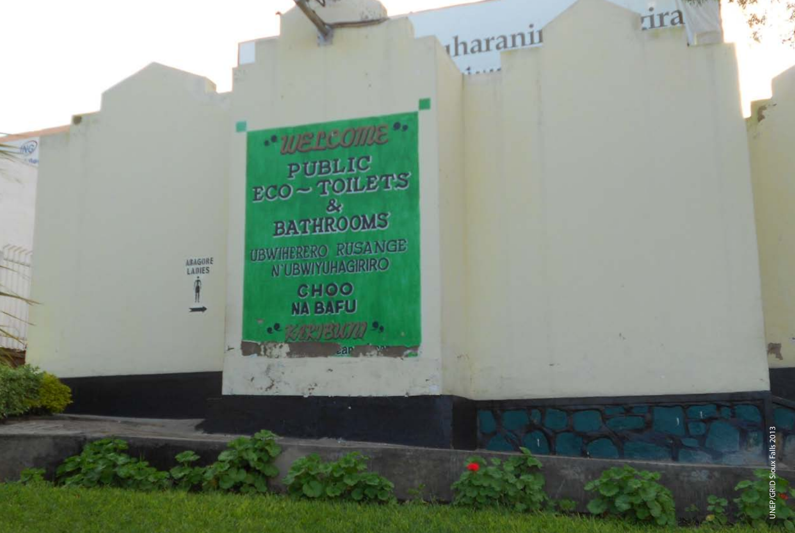
A public eco-toilet in the city centre
