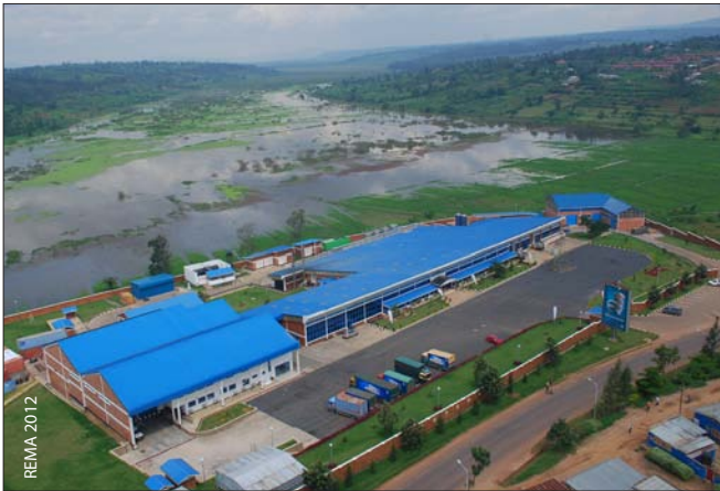
Heavy flooding (shown in this photo; taken after floods in May 2012) caused stagnant water to accumulate near the Inyange Industries and contributed to damage of infrastructure
