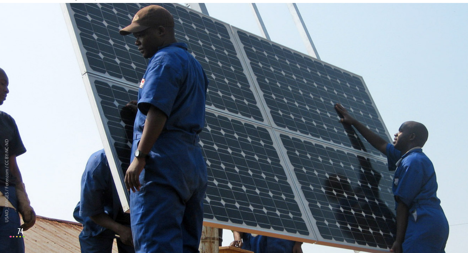
Workers installing solar panels
