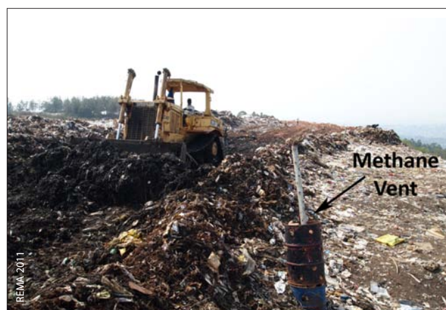
A bulldozer compacting trash at Nyanza near a vent installed to release methane
